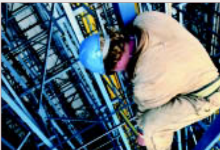
⑤ Structural metalworkers
